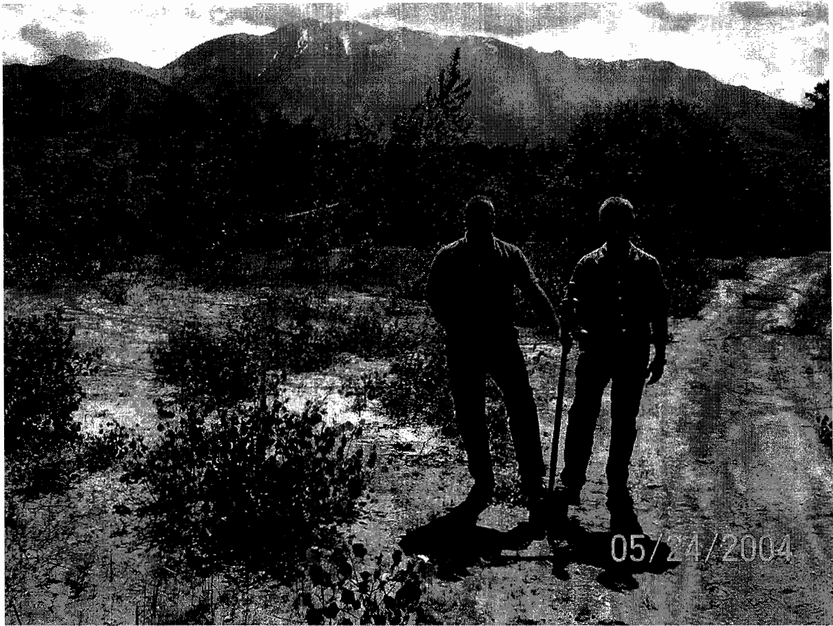
PHOTO 4: GROUND BREAKING FOR THE LFGTE FACILITY (JACK BOYLE, PRESIDENT OF BSE ON THE LEFT AND ERIK COLVILLE OF SCS ENGINEERS ON THE RIGHT)
