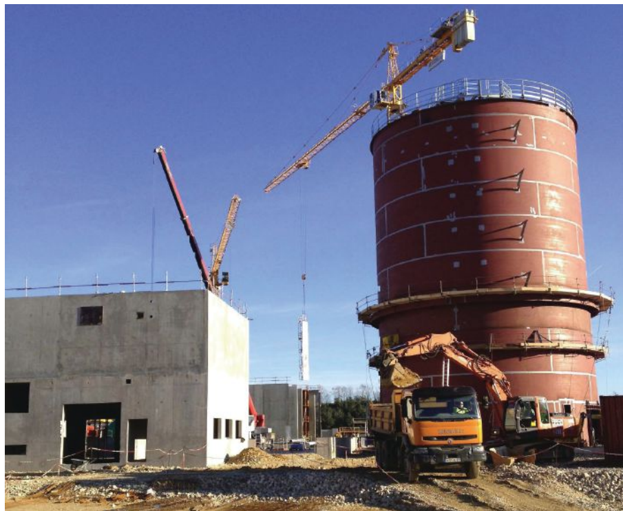
A dry anaerobic digester under construction in Bourgen-Bresse, France
