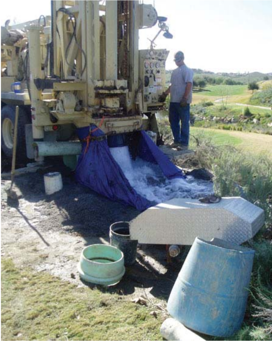
A groundwater supply well is drilled at a golf course in fractured rock terrain in central San Diego County. Abundant groundwater flowed from the well bore during drilling. Photo: Chuck Houser/SCS Engineers
