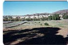
The Cerro Villa Landfill is situated on top of a hill with commanding views and surrounded by high end residential housing.
