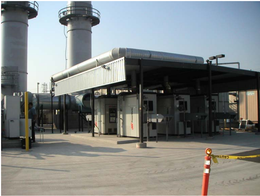
FIGURE 3 - OII MICROTURBINE POWER PLANT
