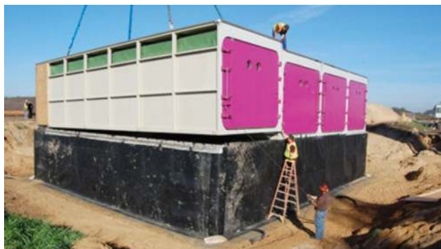
Figure 1: Last of four digesters installed in place. Figure courtesy of Jeff Lindenthal, Monterey Regional Waste Management District, 2013.
