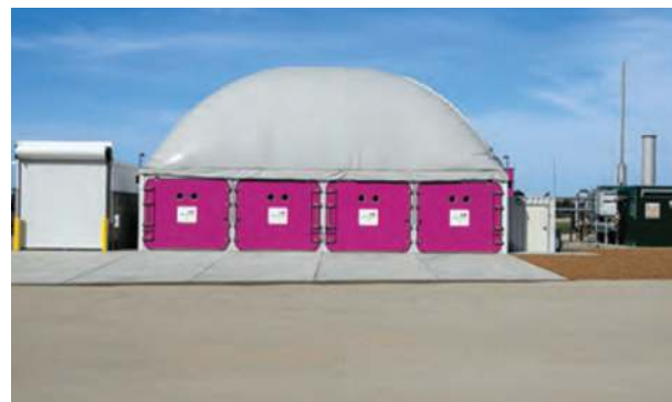
Figure 3: Digester bays of the Marina, CA AD facility. Figure courtesy of Jeff Lindenthal, Monterey Regional Waste Management District, 2013.
