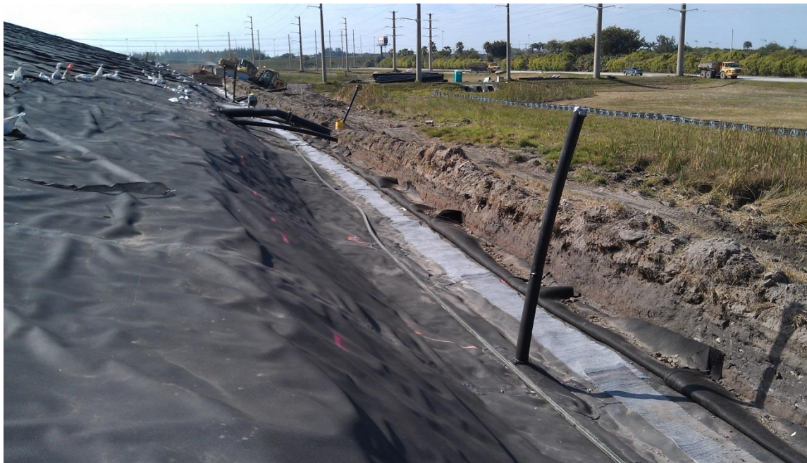
Photo 7. Boot on Vertical Pipe at Cover Geomembrane Penetration
