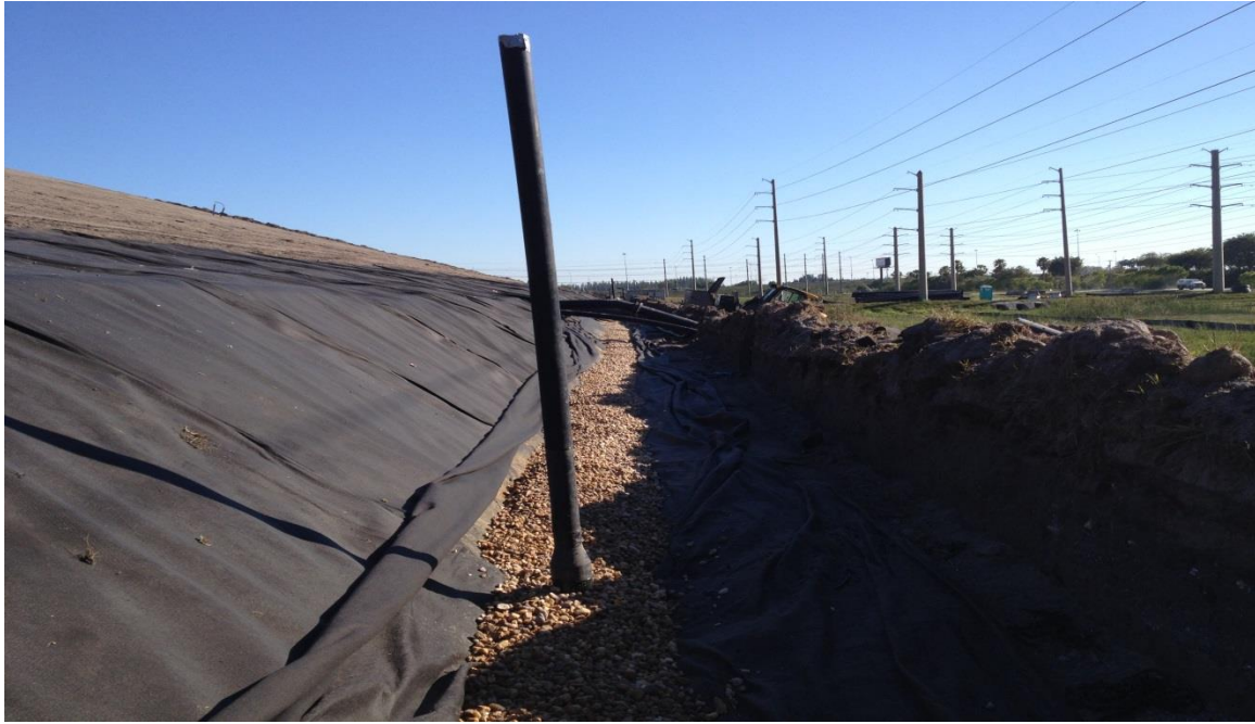
Photo 6. Vertical Pipe for Gas Collection
