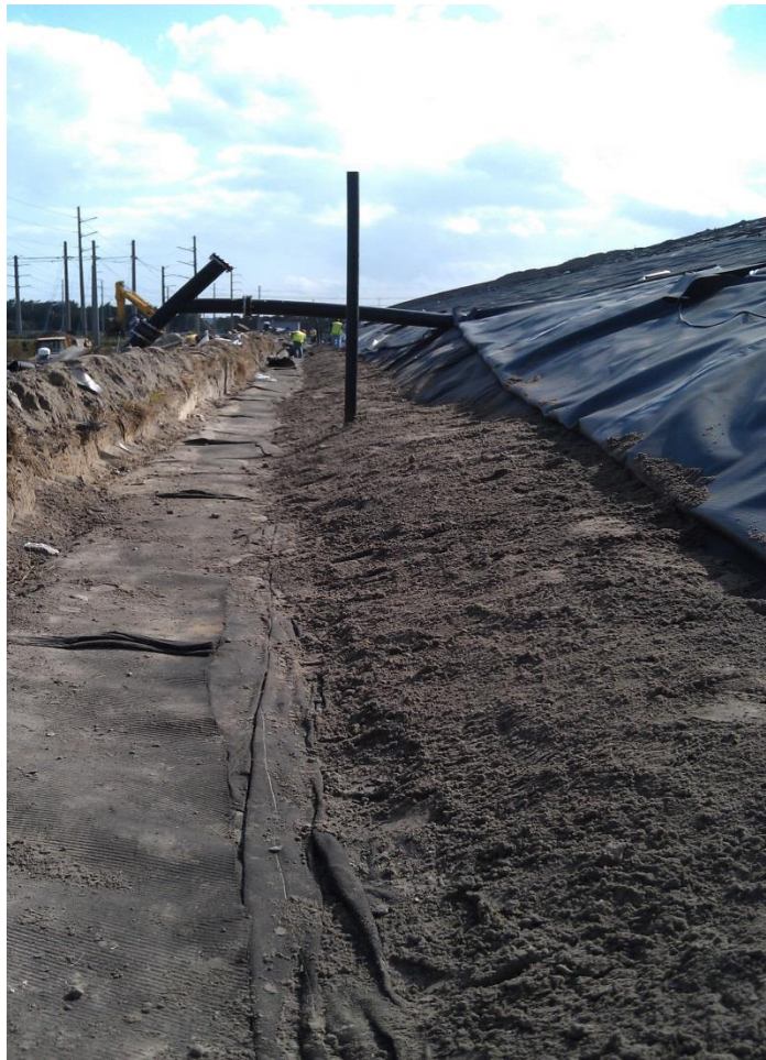
Photo 8. Soil Over LTDS Burrito Before Cover Geomembrane Installation
