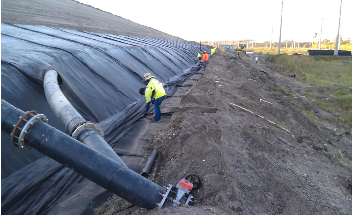
Photo 4. LTDS Burrito Completed
