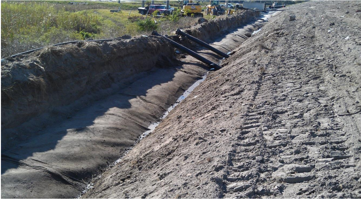
Photo 1. Depression at Toe of Slope
