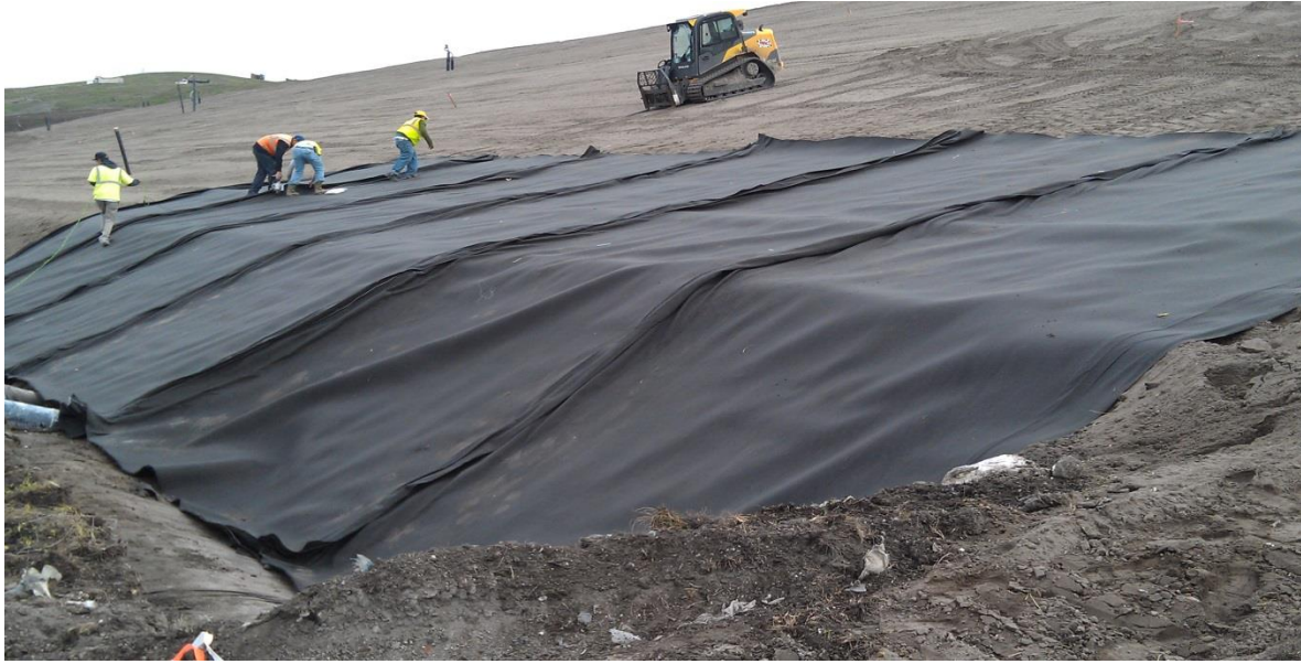
Photo 2. LTDS Geocomposite Over Lower Portion of Slope
