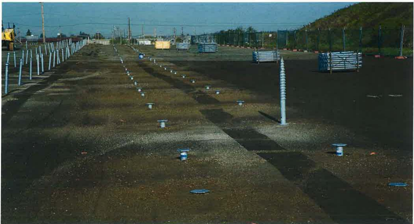
PHOTOGRAPH 8 INSTALLED EARTH SCREWS
