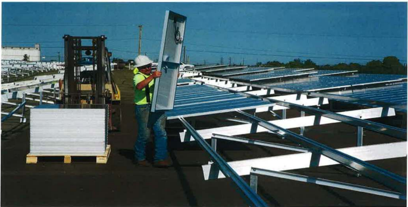
PHOTOGRAPH 10 SETTING SOLAR PANELS
