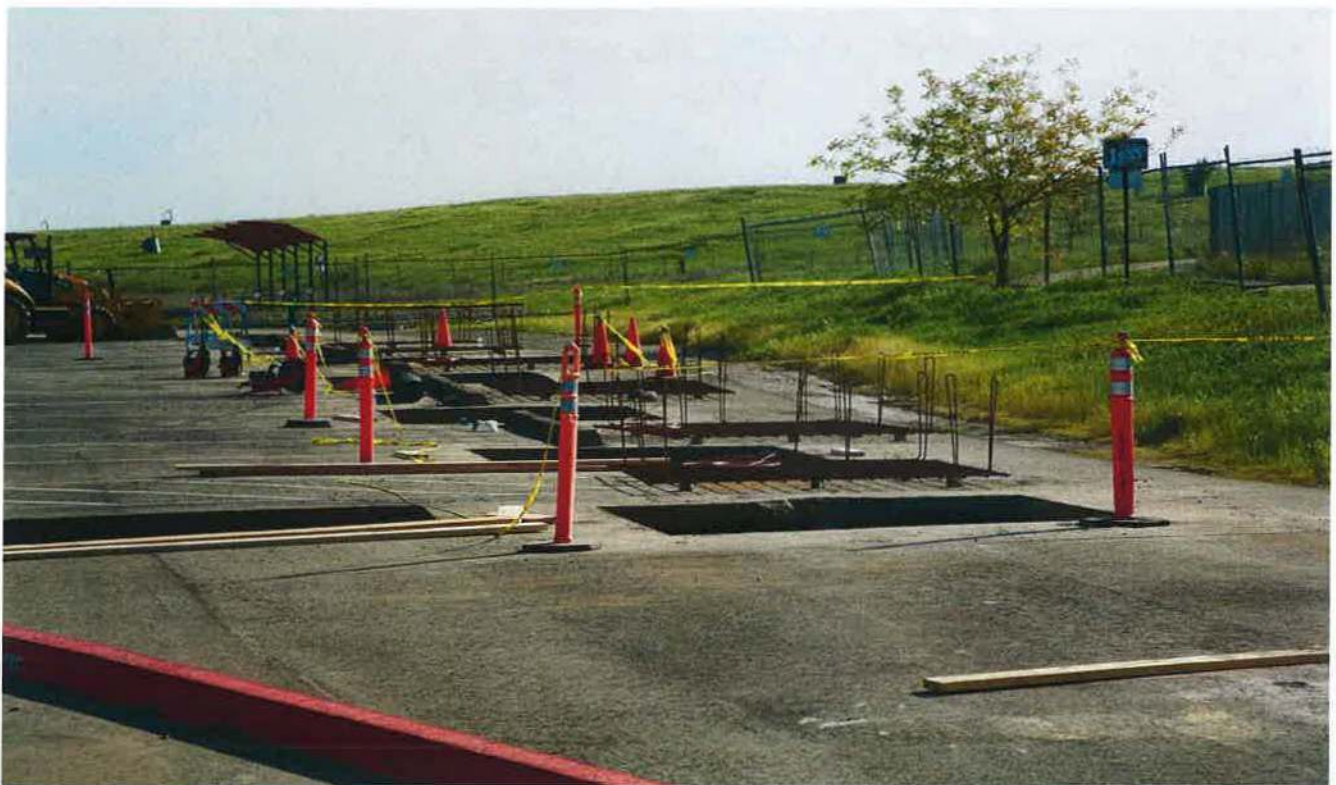
PHOTOGRAPH 2 PARKING COVER FOOTING EXCAVATION
