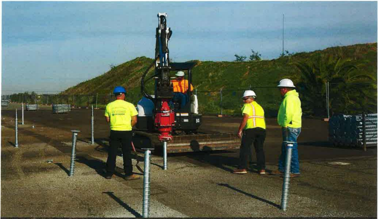
PHOTOGRAPH 7 EARTH SCREW MOUNTS
