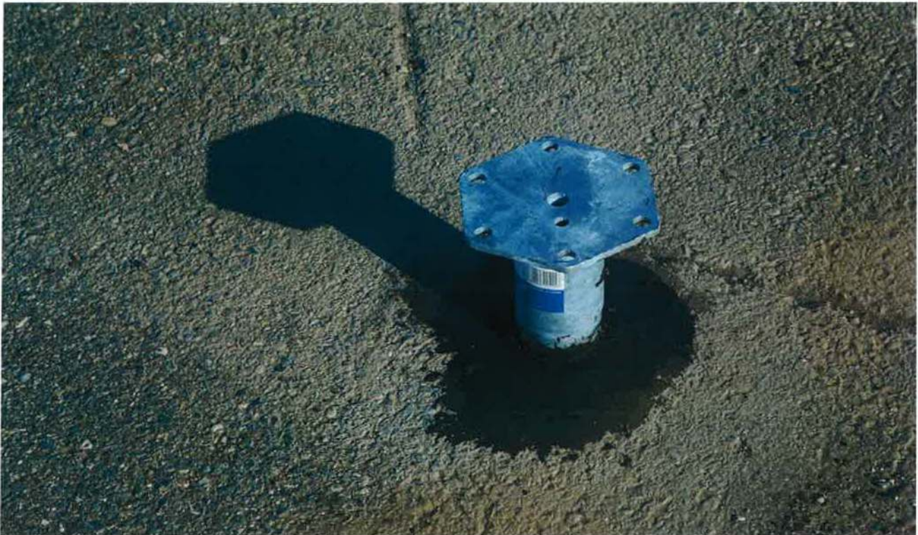
PHOTOGRAPH 9 SEAL AROUND EARTH SCREW
