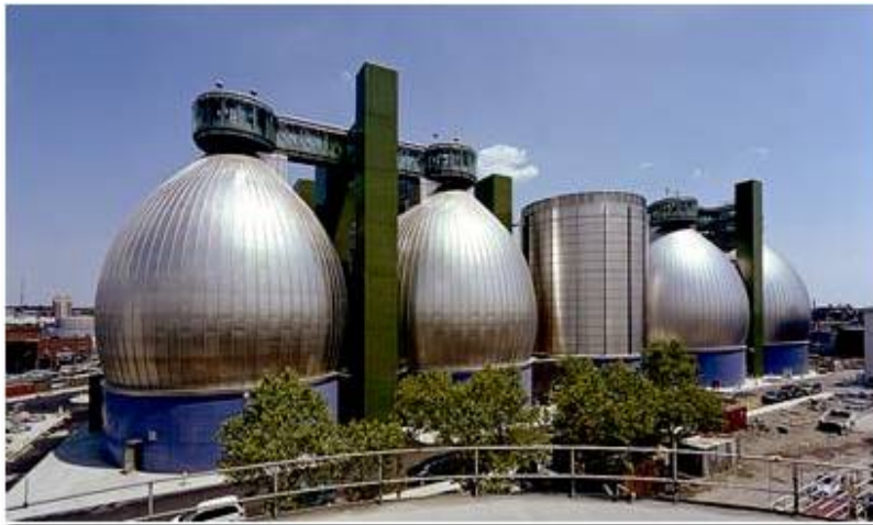
Wastewater treatment plant digester
