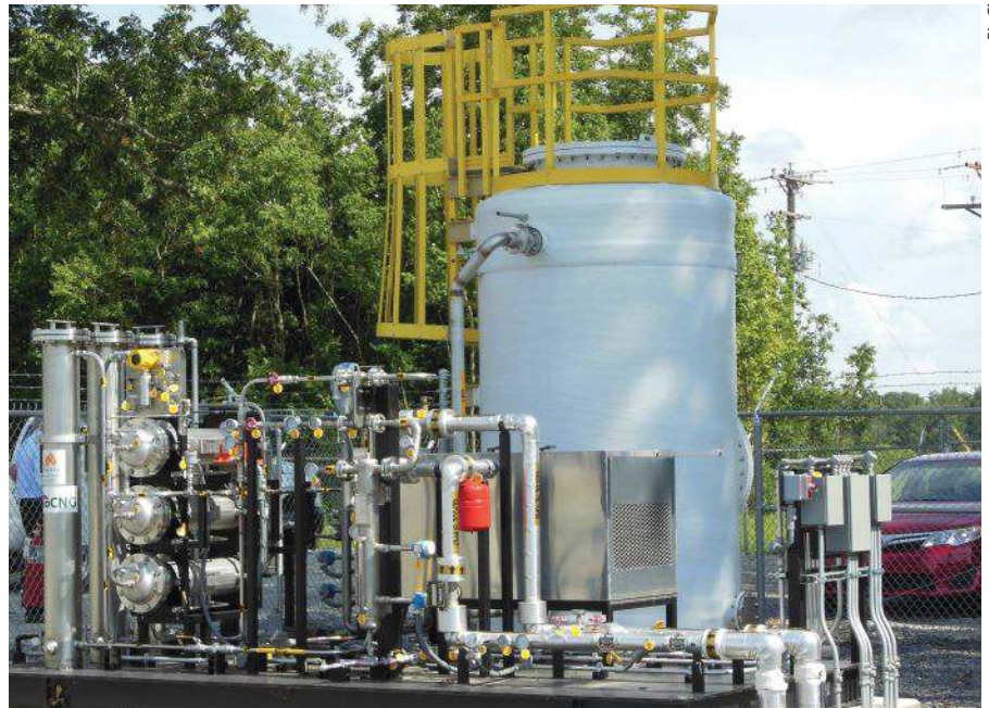
A BioCNG fueling system
