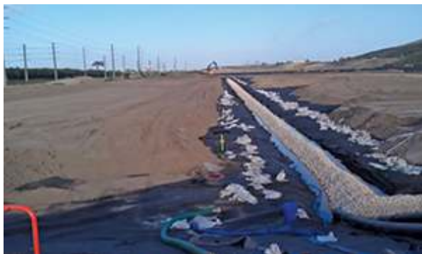
Photo 2. Gravel formed around the pipe.
