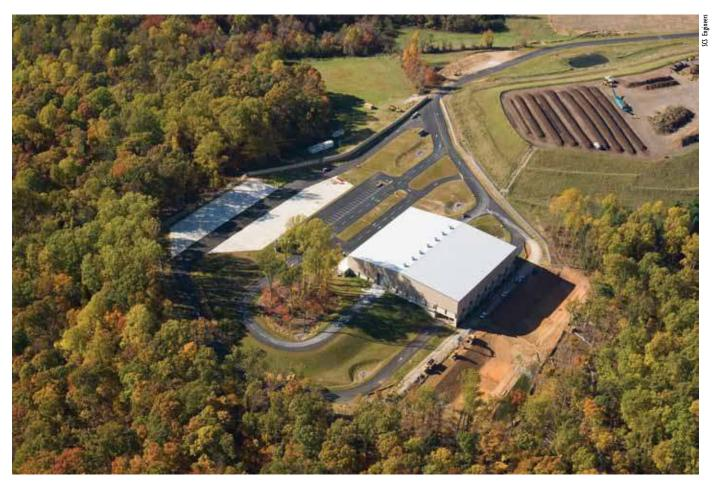
At Frederick County, MD, the transfer station was located on an unused portion of the landfill property adjacent to the composting area that maintained consistency in existing traffic routes onsite and siting the building along a hillside to take advantage of natural grades to accommodate the full depth tunnels.
