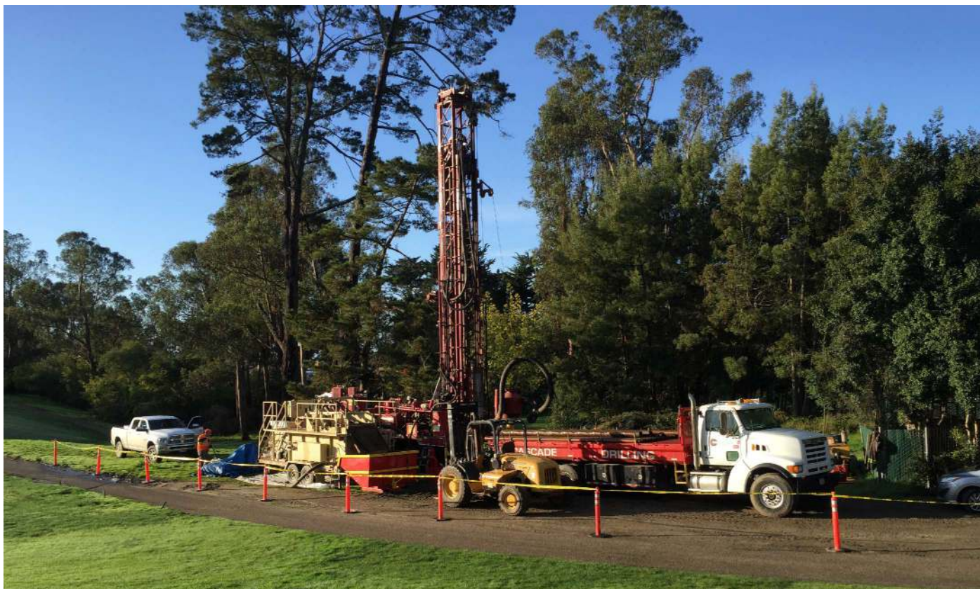
A drilling rig in coastal central California. Installing a supply well for groundwater requires about 100 square feet for the well, as well as room to navigate a 35-by-10-foot truck and sufficient clearance to raise a 35-foot drilling mast. Photo by Chuck Houser
