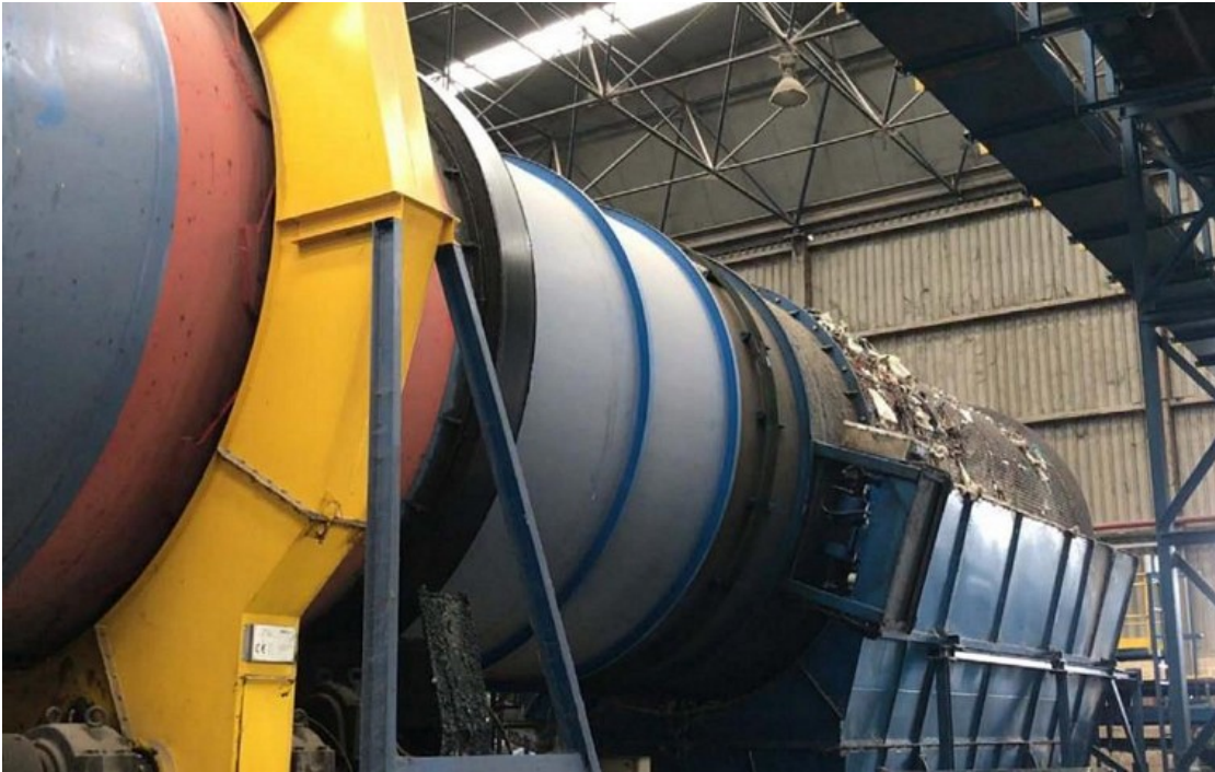
An MSW drum pulper in operation, in Spain.
