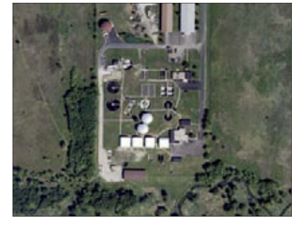
PROFILE: Village of Bartlett Wastewater Treatment Plant
