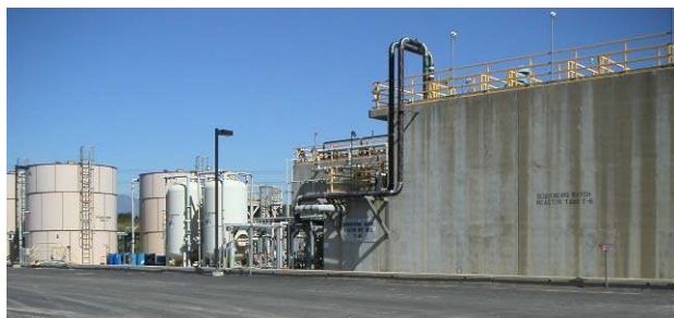
Figure 1 – Leachate Treatment Plant (LTP)
