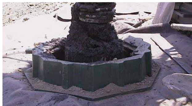
Figure 5 – Drilling in Saturated Refuse
