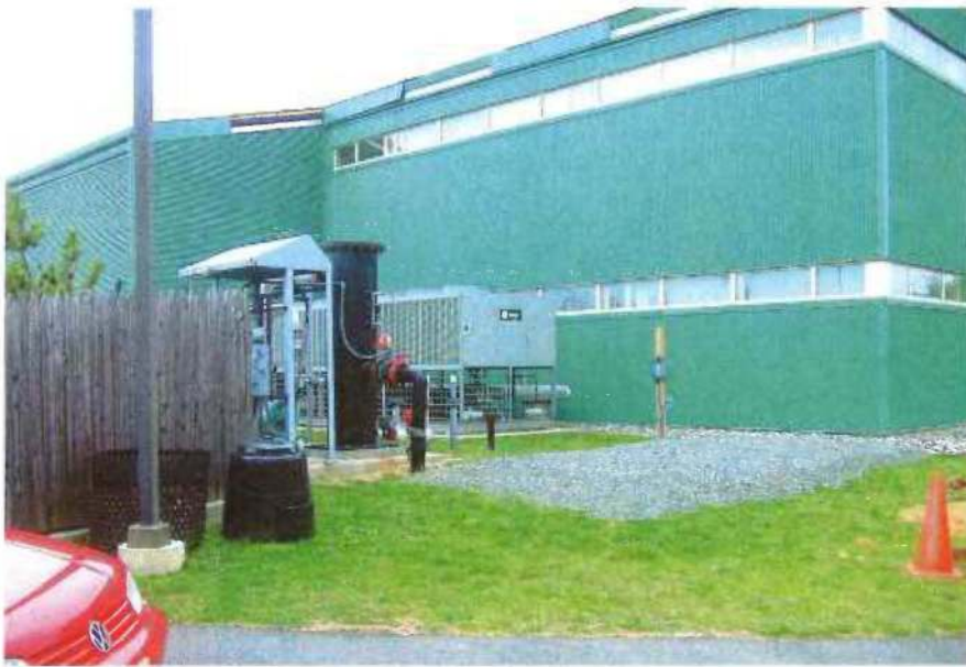
SKID ROW: A landfill-gas-to-energy skid at the Rutgers University EcoComplex in Newark, N.J.
