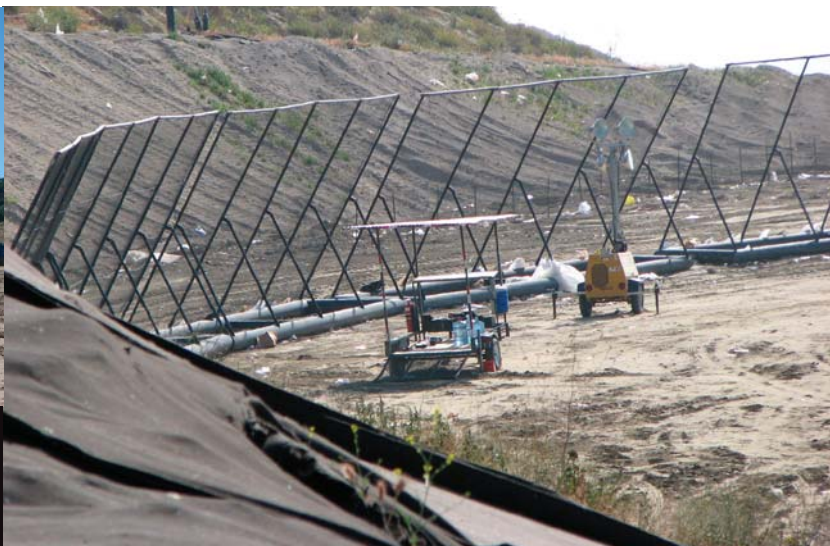
FENCED IN: Portable litter fencing is in use throughout the country to prevent blown landfill litter from being carried off site.
