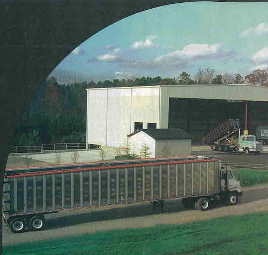
ELEVATE: If open-top trailers are going to be used to transport waste, a sloping site or the grading of a flat site is needed for a transfer station.
