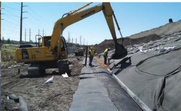
Photo 6: The pipe is encased in gravel.
