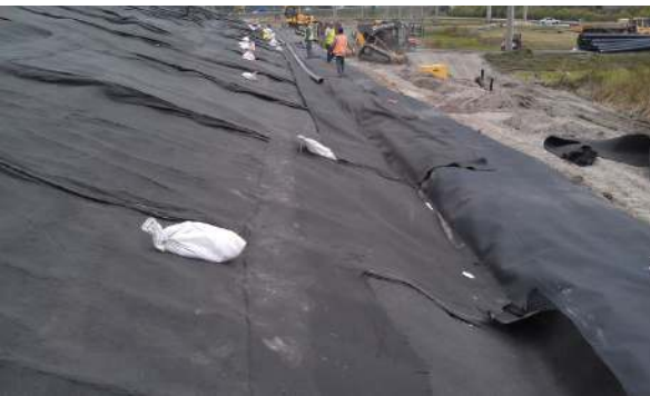
Photo 5: The RTDS geotextile and pipe are positioned.
