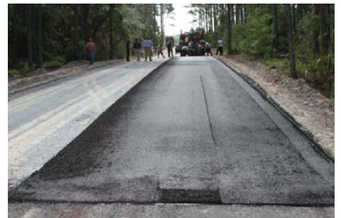
"Ash-fault" roadway construction
