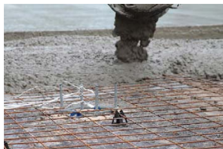
Instrumentation placed in concrete slab
