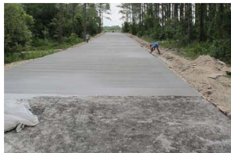
Control and "Ash-Crete" roadway test sections
