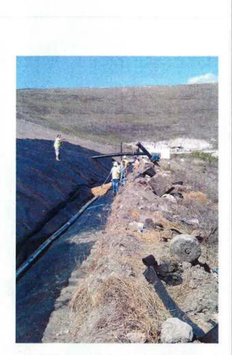
The LTDS geocomposite is anchored on the slope approximately 10 ft. to 15 ft. above the perimeter berm. After installation, the cover geomembrane comes in contact with the LTDS geocomposite, and the geocomposite becomes the sole conduit for liquids below the cover geomembrane flowing to the bottom of the slope.
