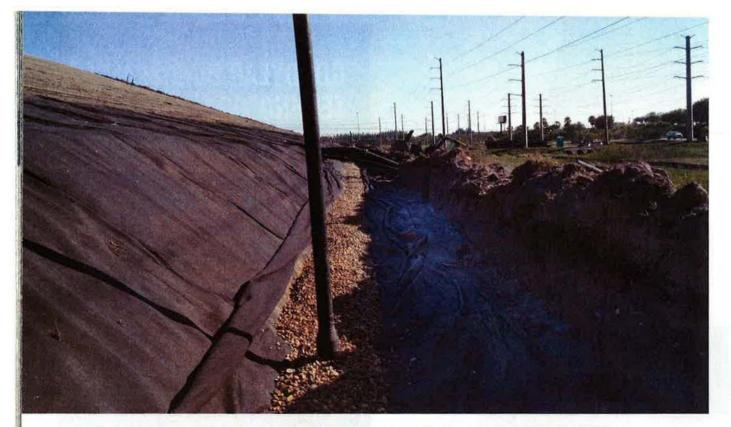
final cover is constructed over the slope above the LTDS at a later date. In that case, the LTDS geocomposite will be placed above the LTDS burrito; therefore, measures must be taken to ensure that no soil is trapped between the LTDS geocomposite and the LTDS burrito that could potentially create a future bottleneck in the flow path of leachate to the LTDS burrito.
