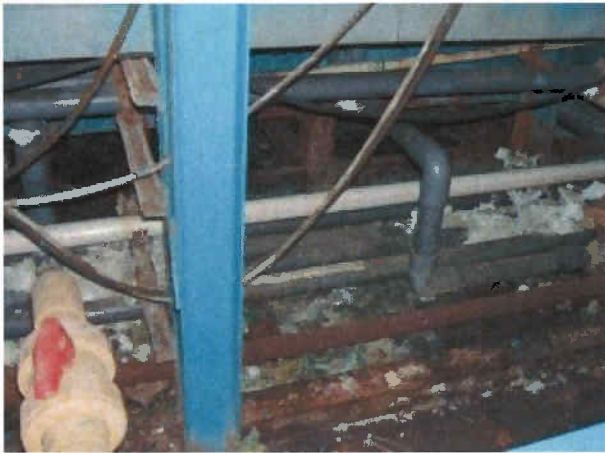
Figure 1: The concrete floor beneath the plating operation was visibly corroded and in poor condition.
