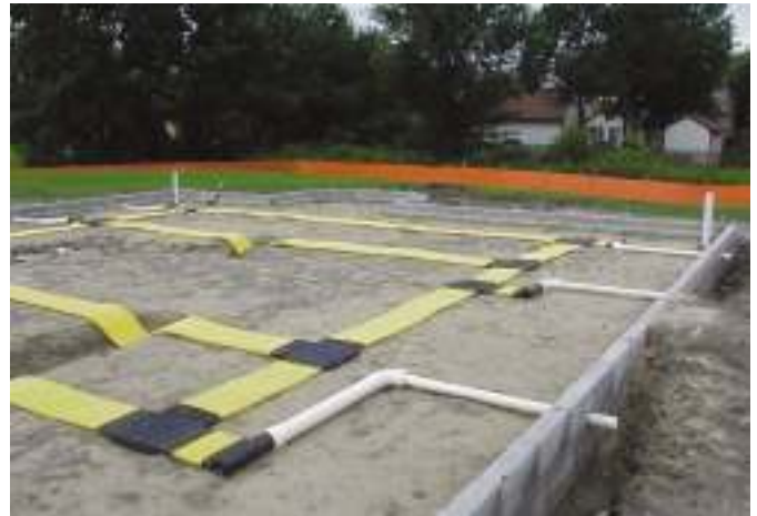
ABOVE LEFT A passive system with a PVC membrane barrier at a building site of single-family houses ABOVE RIGHT Foundation vents
