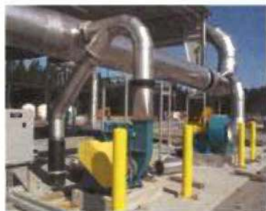
An aeration unit
