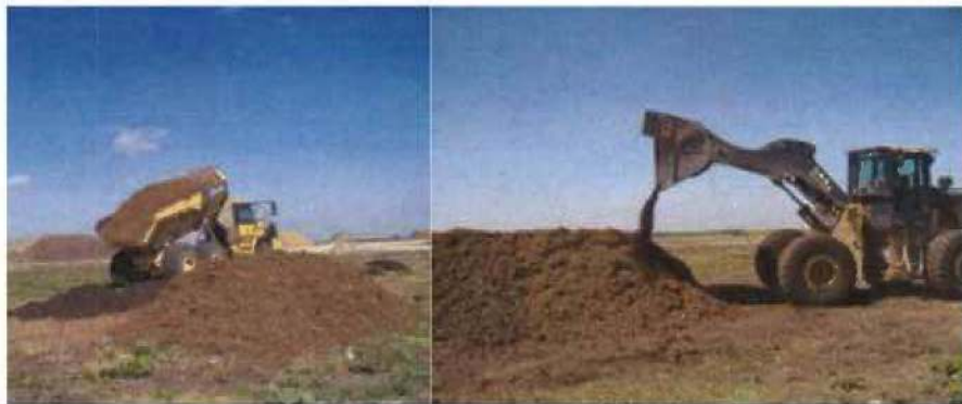
Piles of yardwaste and biosolids are prepared for the mulching process.
