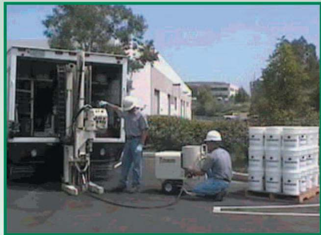
On-site direct injection of ORC
