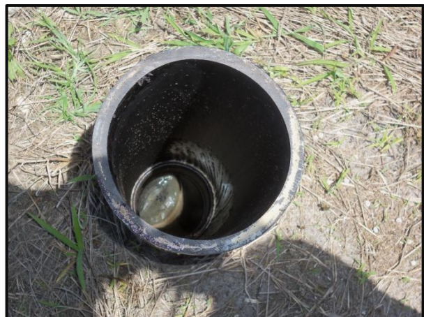
WELL WITH WATER IN LATERAL; HOWEVER, THE MAJORITY OF WELLS AT BEE RIDGE WERE DRY IN THE MAY 2014 FIELD INVESTIGATION.
