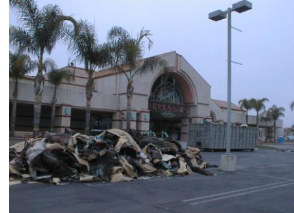
SCS assisted in successfully diverting 97% of the C&D materials generated during the deconstruction of a multiplex theater.
