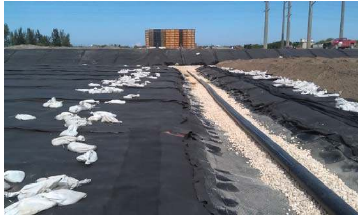
Photo 1: Gravel placed below pipe
