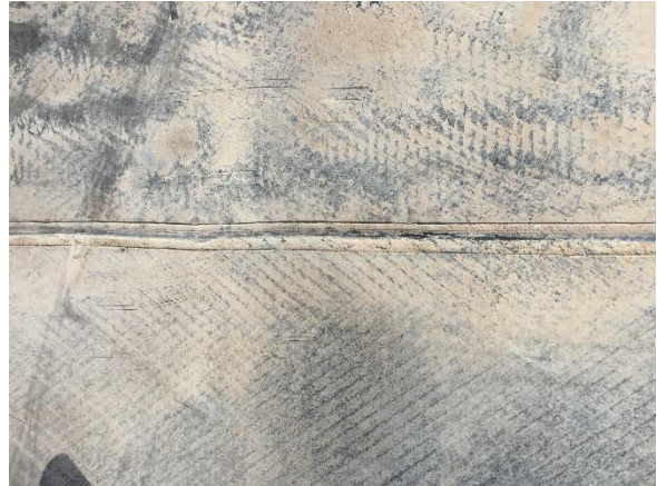
Figure 3(b). HDPE geomembrane Sampling
