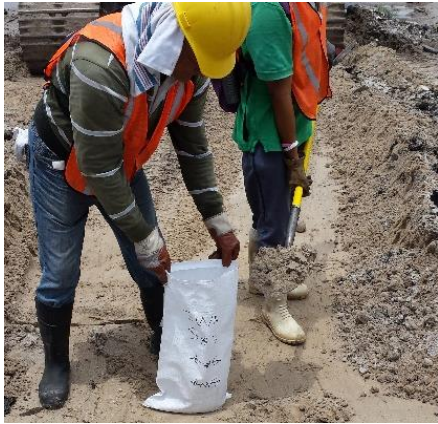
Figure 1 (a). Granular Drainage Layer Samples
