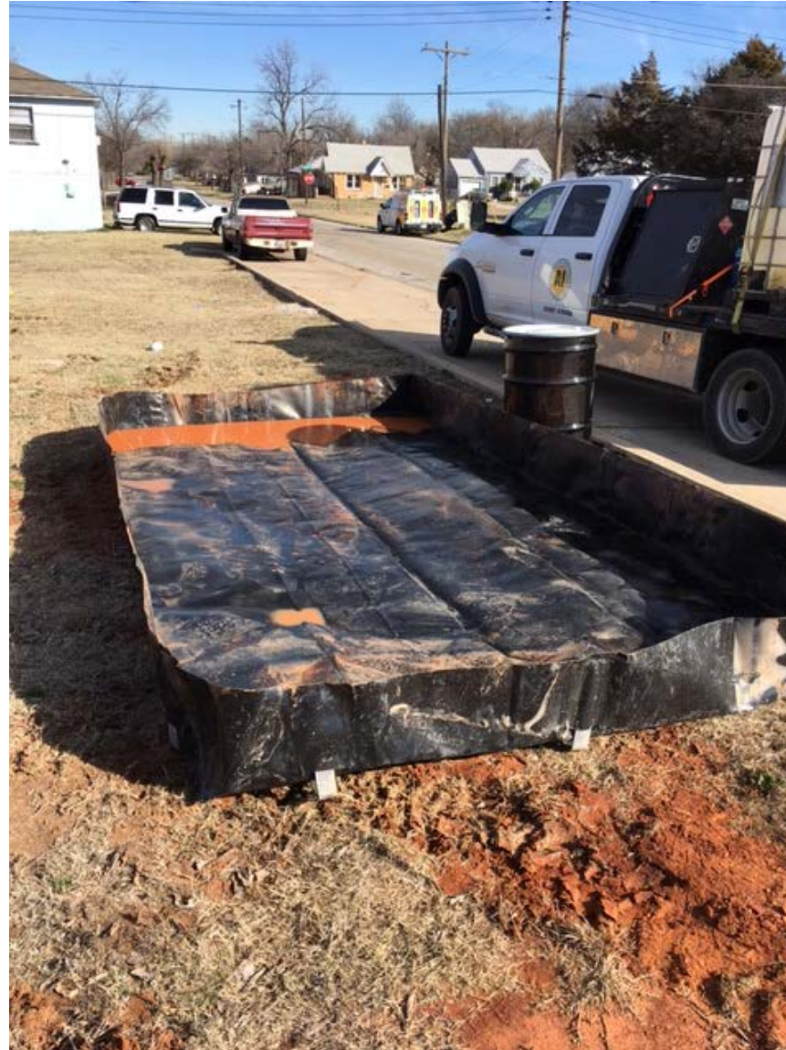
Portable decontamination pit
