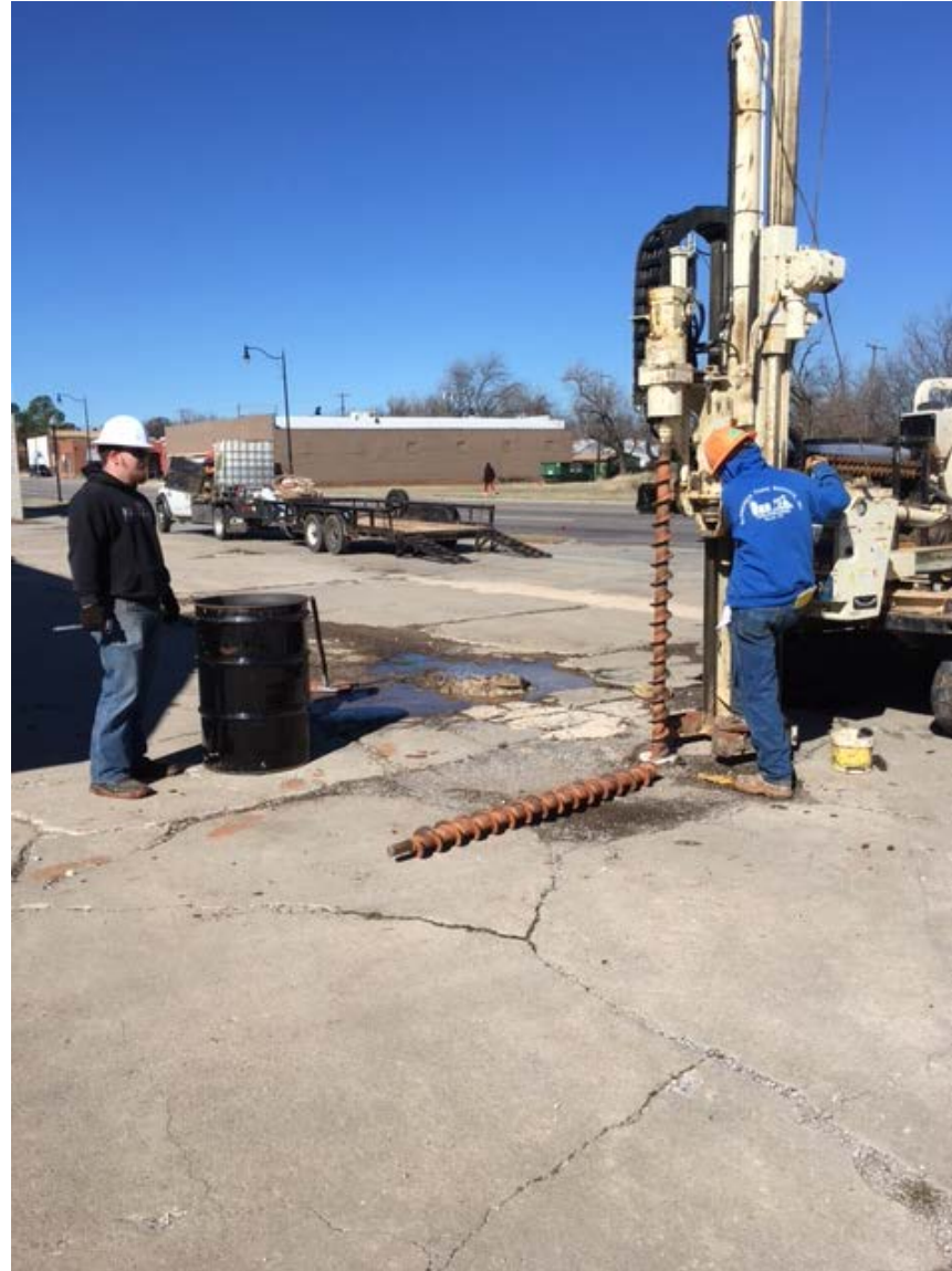
Solid-stem drilling at SB-05 near possible tank pit area
