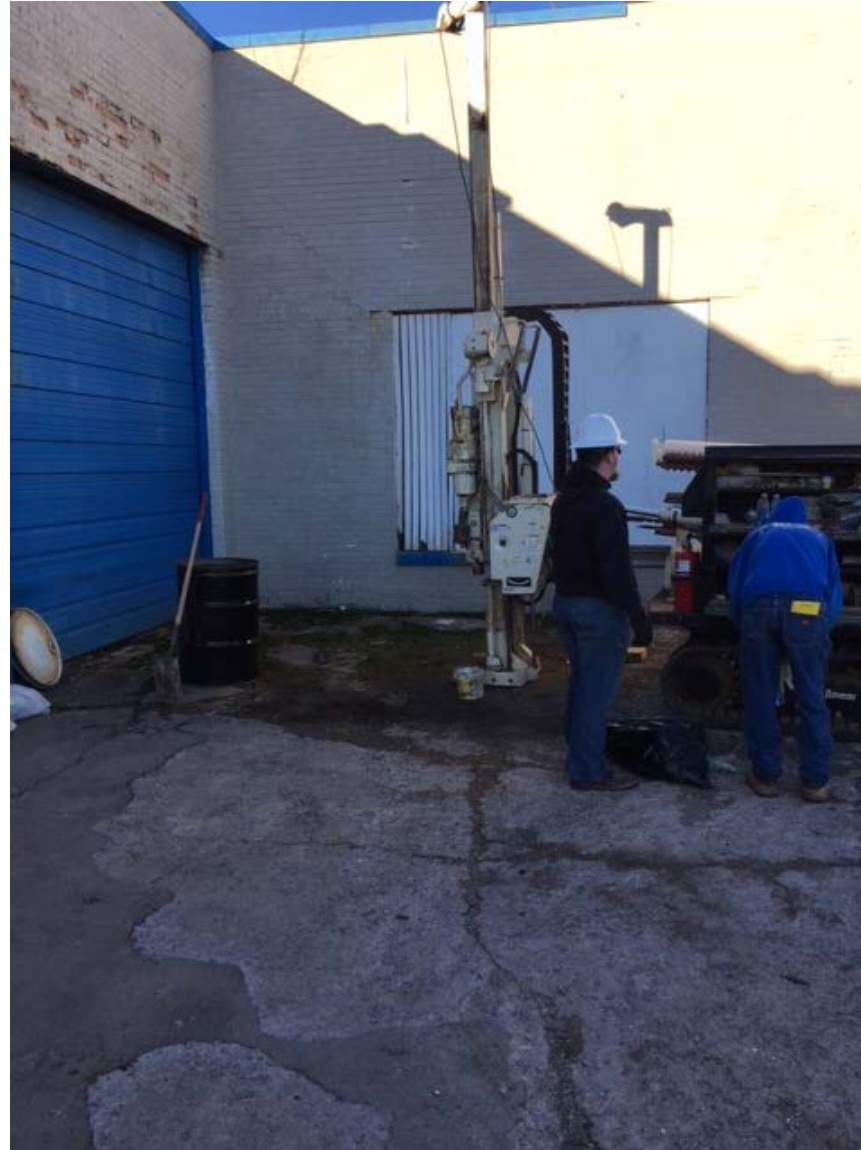
Geoprobe set up at SB-04
