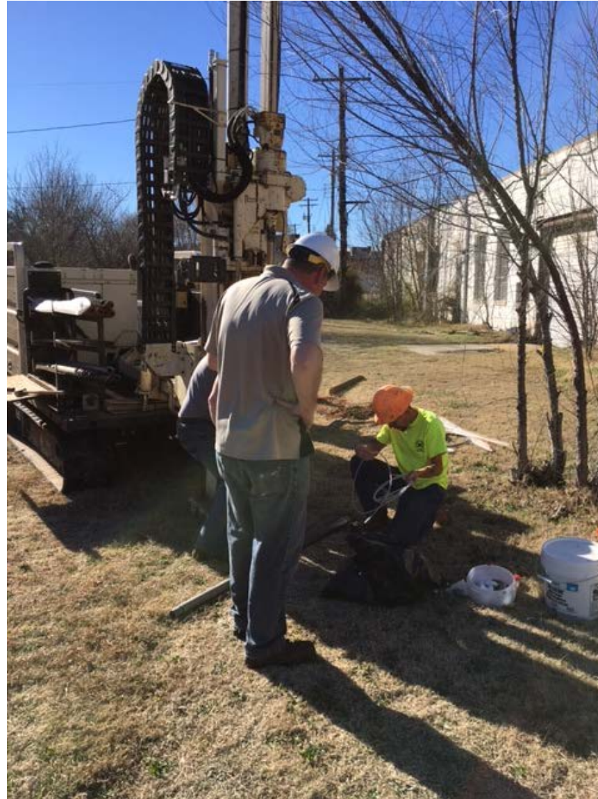
Subsurface vapor implant installation at SV-05
