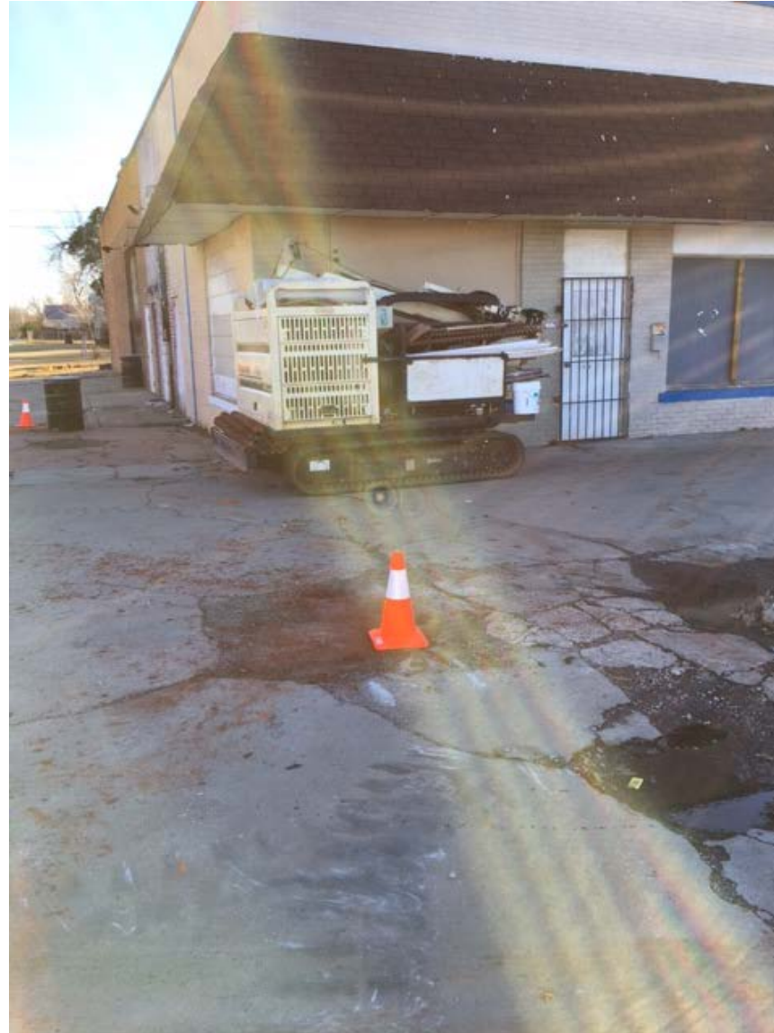
Geoprobe setting up near SV-03 location near building
