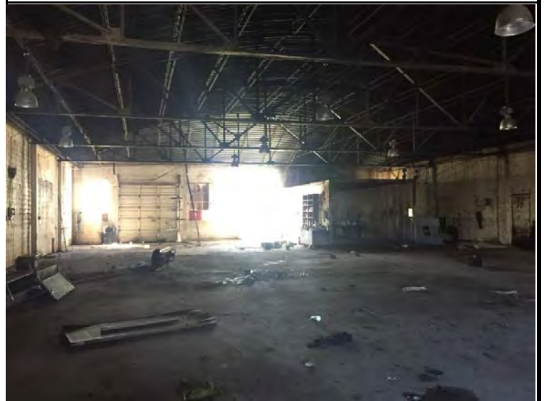
Photo 4: Room 11 - Asbestos Containing Window Pane Caulk
