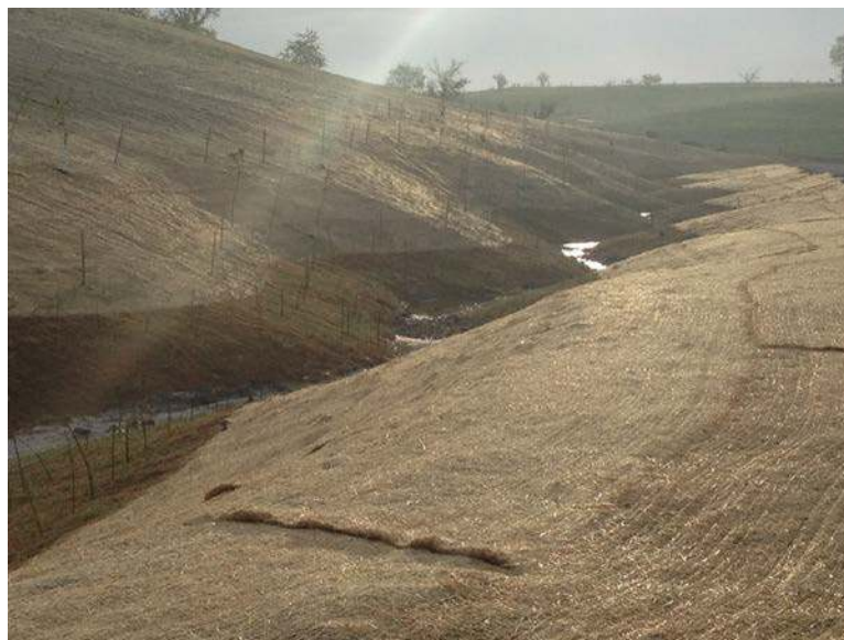
Figure 6. Stream mitigation area after initial construction.
