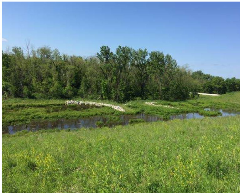
Figure 5. Completed wetland mitigation area.
