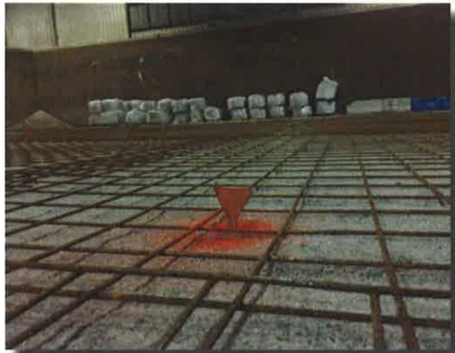
Figure 5: Floor wear indicator. Photo courtesy of Cornerstone Construction, Orlando FL.
