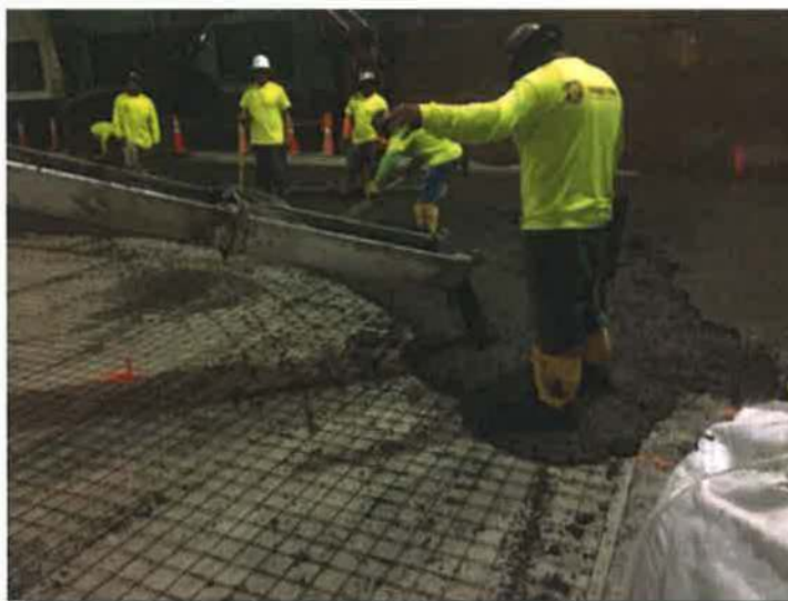
Figure 3: Pouring a topping with hard mineral aggregate.
