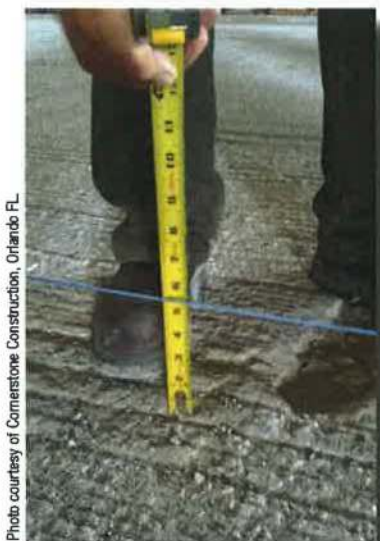
Figure 2: Start of repairs – grinding existing concrete.
