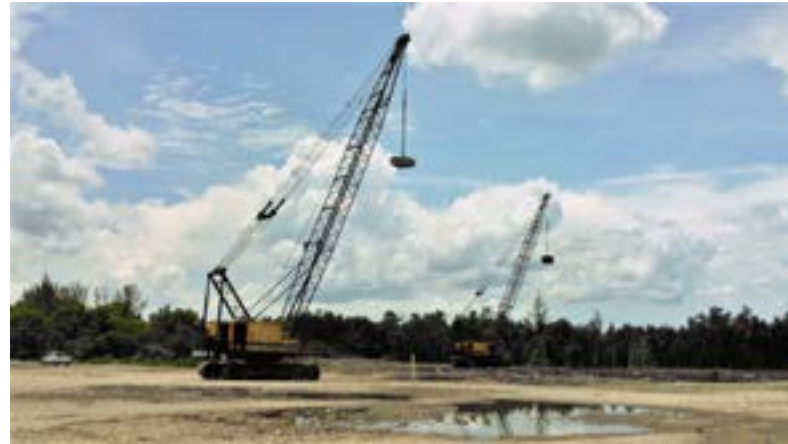
Figure 1 - Dynamic compaction crane and weight.
