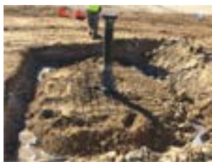
Well bore reinforcement gate
