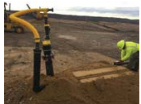
Checking slope on lateral
