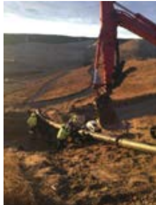
Fusion of 12-inch HDPE SDR 17 header
