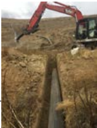
Trench for road crossing
