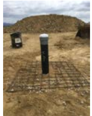
Completed single landfill gas extraction well
