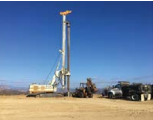
Setup for drilling
