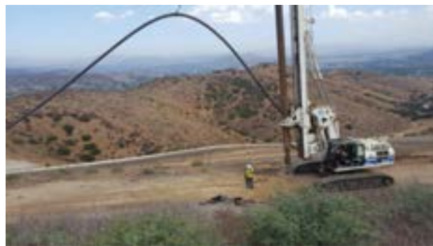
Setting of HDPE well casing
