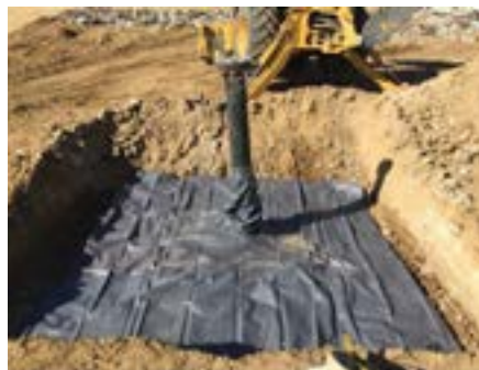
Geomembrane skirt with boot
