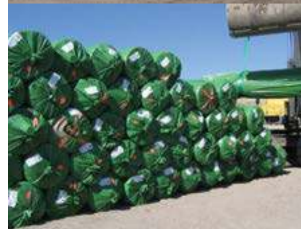
Rolls of GCL being unloaded at project site.
