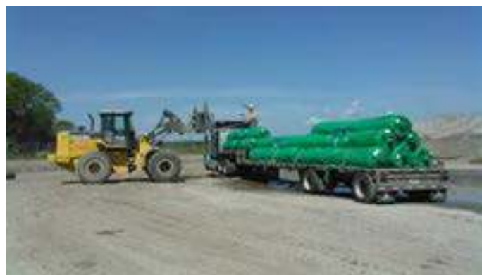
Rolls of GCL delivered to project site.
