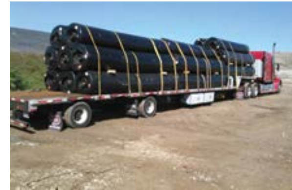
Rolls of geotextile delivered to project site.
