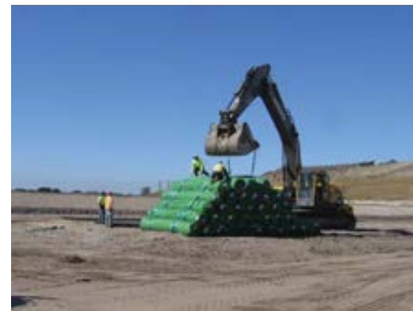
Rolls of geotextile delivered to project site.
