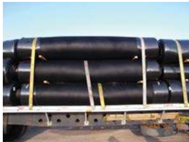
Rolls of geomembrane delivered to project site.
