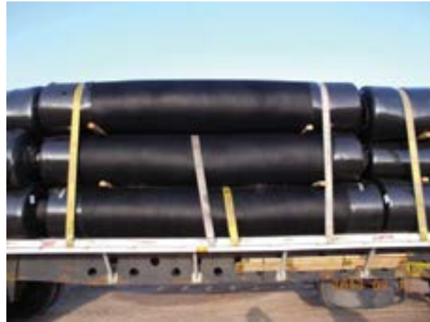
Rolls of geomembrane delivered to project site.
