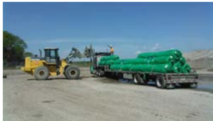
Rolls of GCL delivered to project site.
