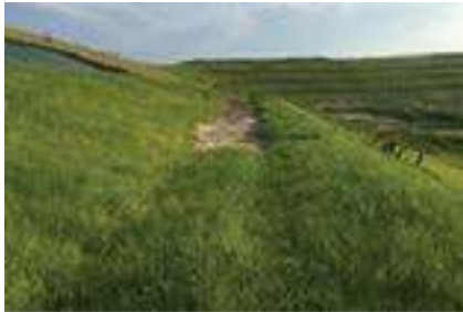
Figure 2: Landfill bench and well-vegetated side slopes with easy access to landfill gas well near the bench
