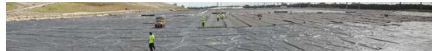
Geocomposite drainage layer installation above geomembrane.
