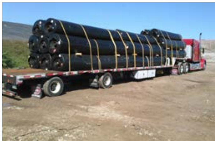
Geocomposite drainage material delivered to site.
