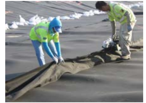
Sewing of the upper geotextiles of adjacent geocomposite panels.
