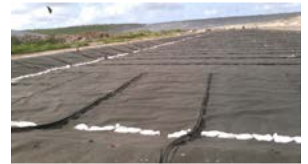
Geocomposite drainage layer in place.
