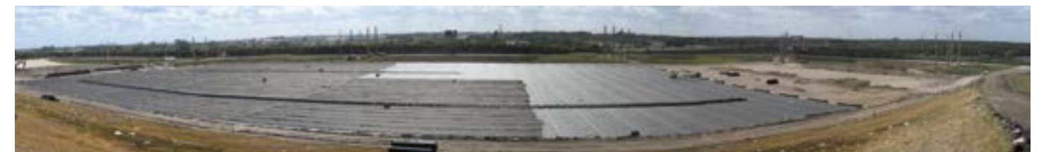
Installation of geocomposite in progress.
