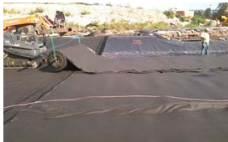
Geocomposite drainage material during installation.
