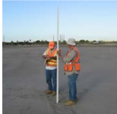
Cell base area under construction with specified slopes.
