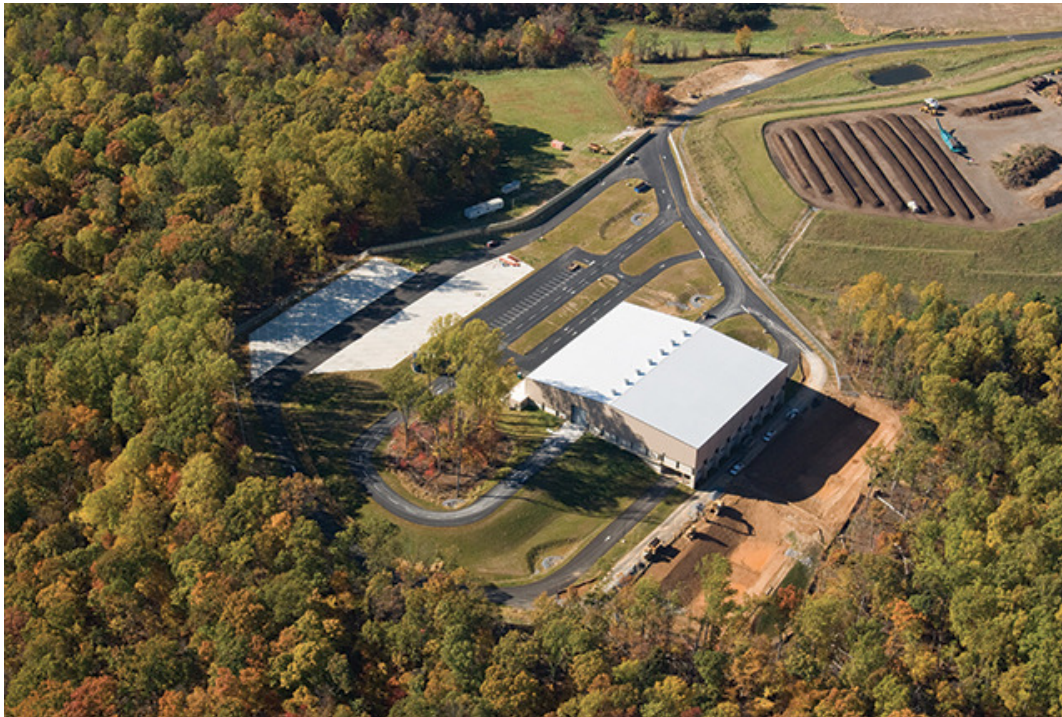
Transfer station designed by SCS Engineers SCS ENGINEERS
