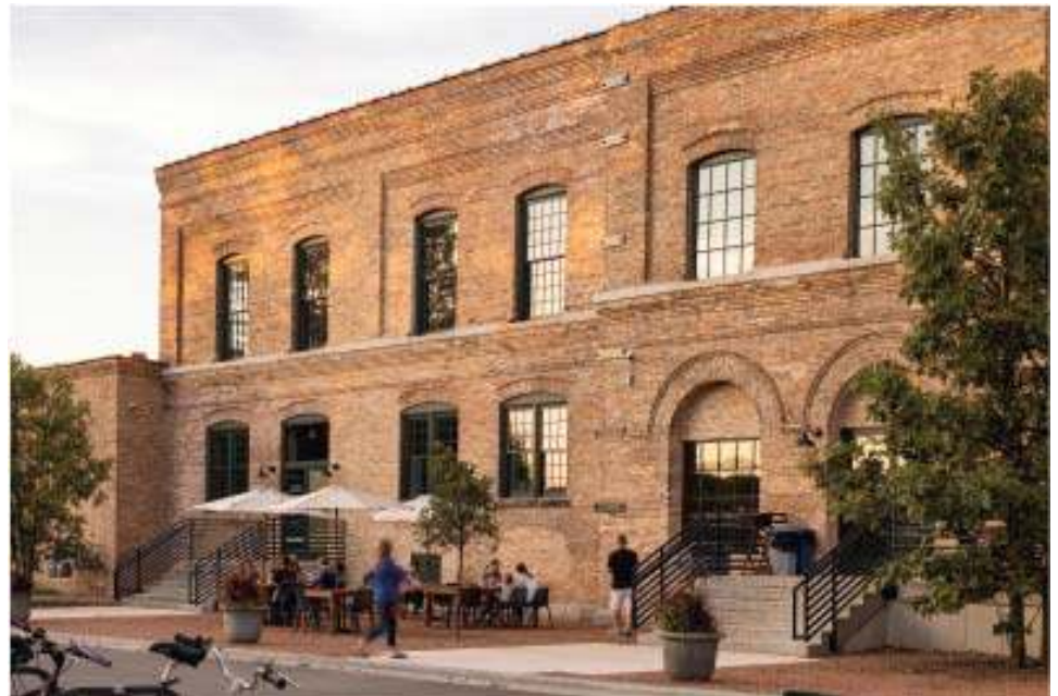
The different sides of Garver: The refurbished brick that visitors see on the exterior of the renovated Garver Feed Mill building was reclaimed from a local source — the former French Battery building at Union Corners. The entrance (lower left) features a combination of reclaimed steel and railroad rods.
