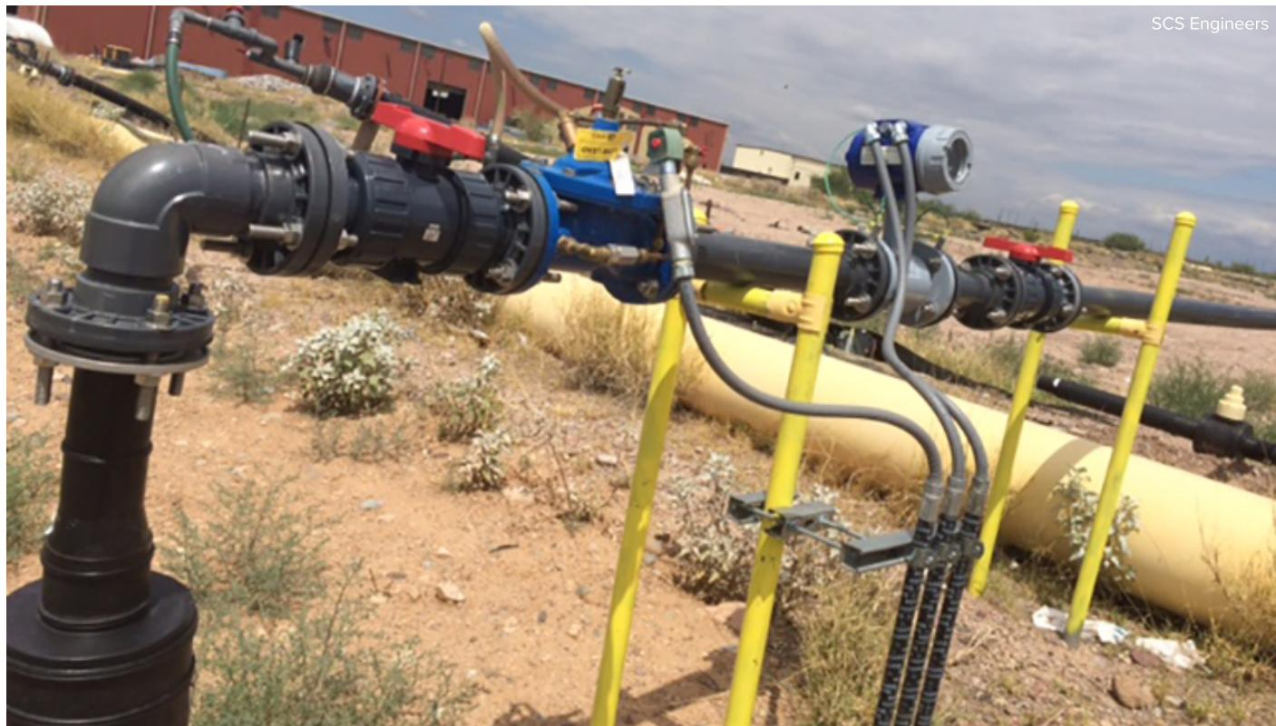
He and those in his industry have found limits to how much liquid can be added; tipping that balance can lead to outbreaks on side slopes, stability issues and odors.
