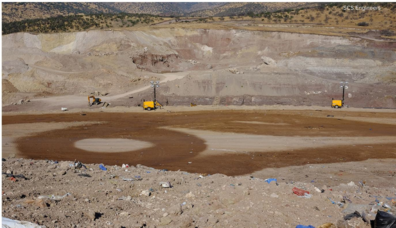
A research and demonstration project at Northern Oaks Landfill in Harrison, Mich., yielded successful results: a moisture content of 35 percent was achieved with horizontal leachate injection/recirculation pipes. Laying the pipes on top of the compacted waste enhanced lateral movement of leachate.
