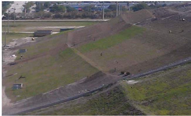
Photo 2 - Tack-on berms and swales on landfill final cover.
