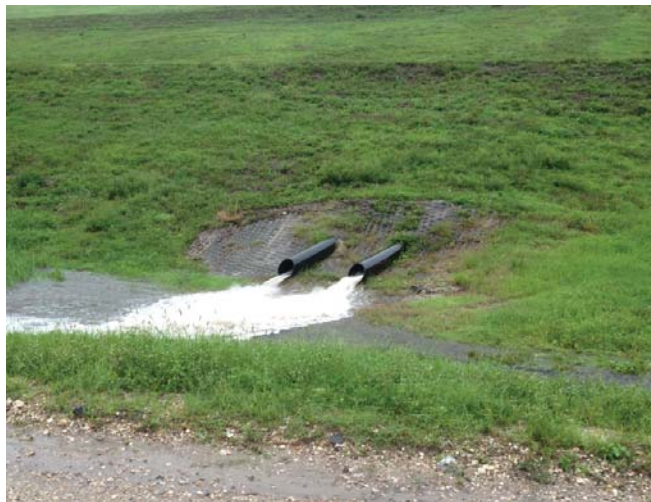
Photo 3 - Discharge points of downchute pipes.
