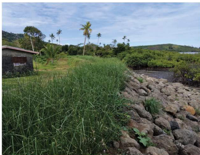
Fig. 5. Vaidogo village NbS seawall.
