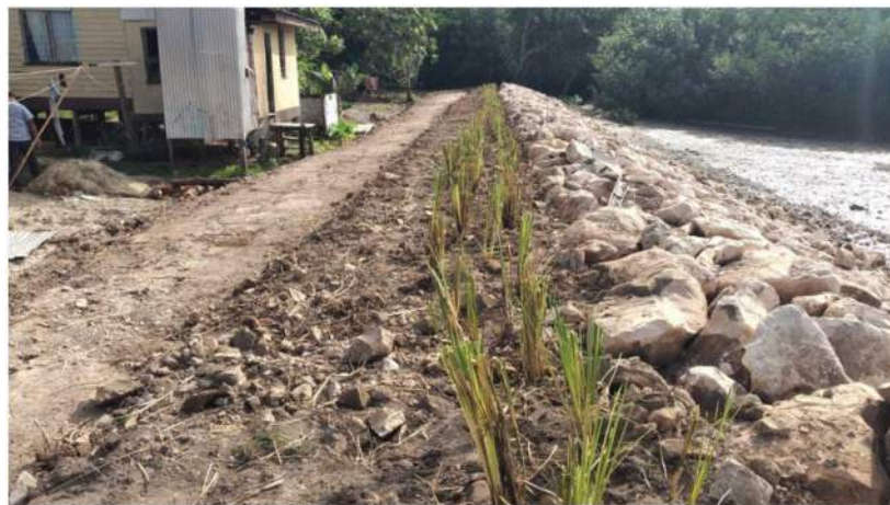
Fig. 4. Nabubu village NbS seawall.
