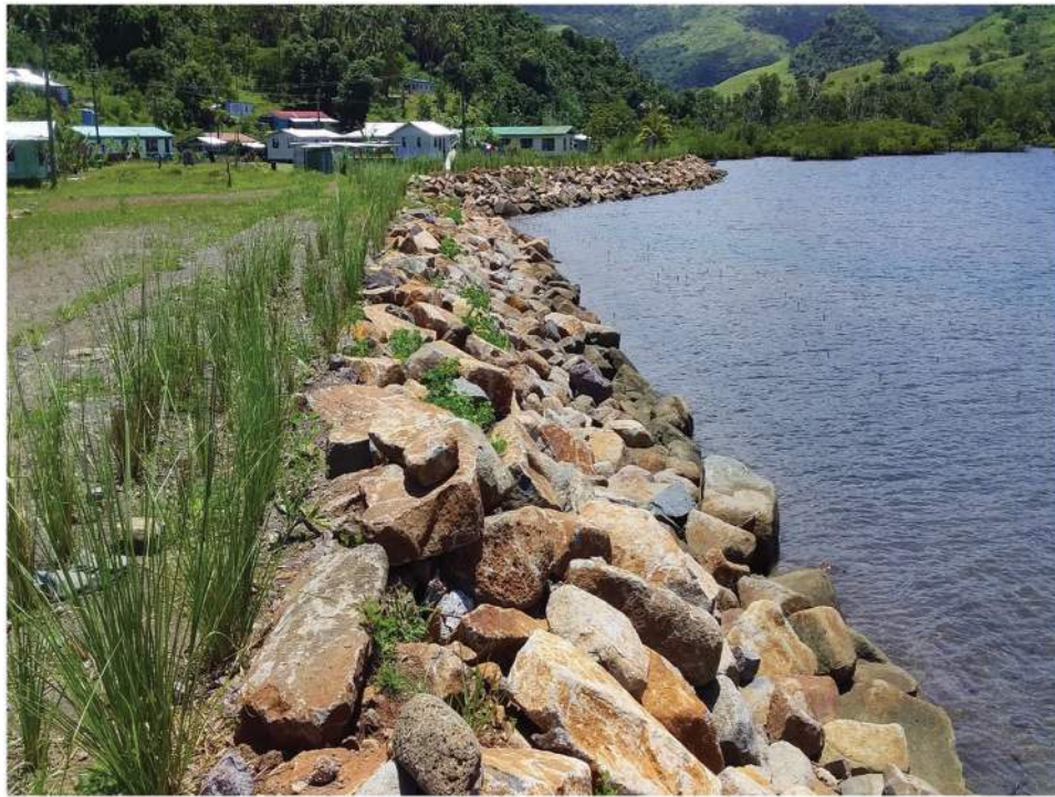
Fig. 6. Nabukadra village NbS seawall.
