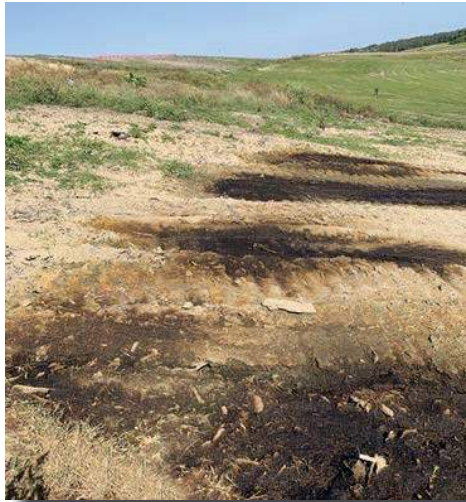
Figure 1: What appear to be shadows in the images are seeps of dark leachate.
