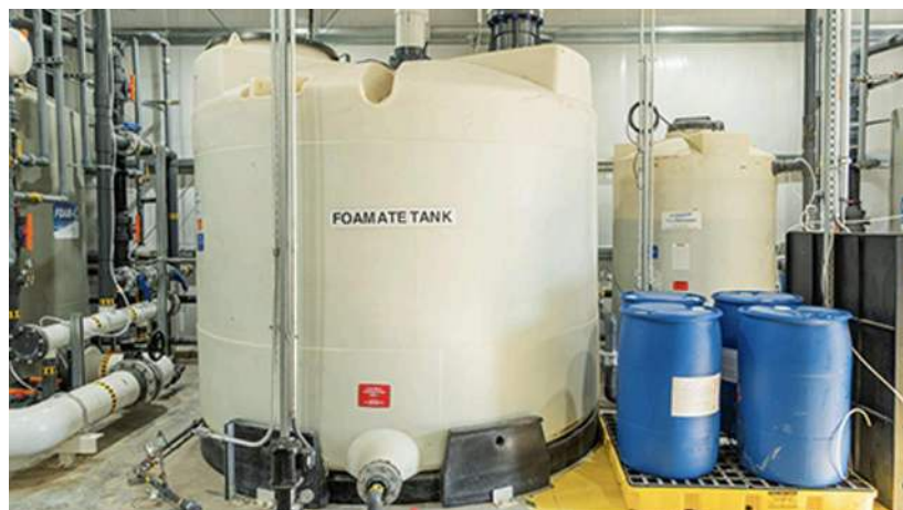
4) A foamate tank with collected PFAS is where the bubbles in the foam pop and return to a liquid state.
