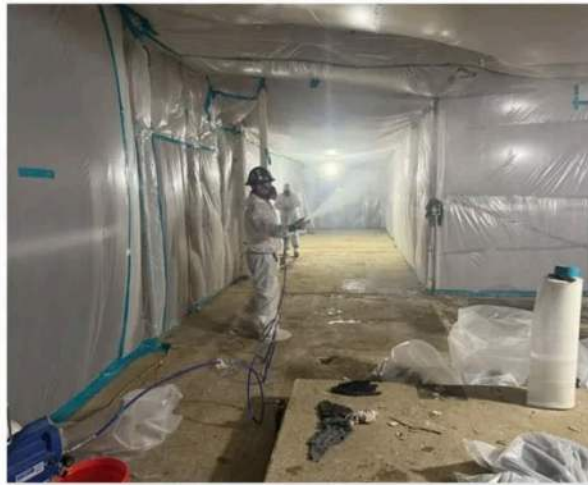
Crews work to remove asbestos-containing materials from a commercial building that will be converted into residential.
