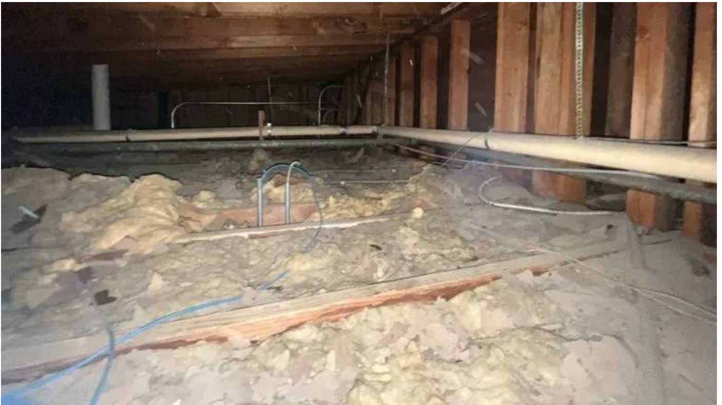
Credit: SCS Engineers in Las Vegas/Henderson, Nevada
