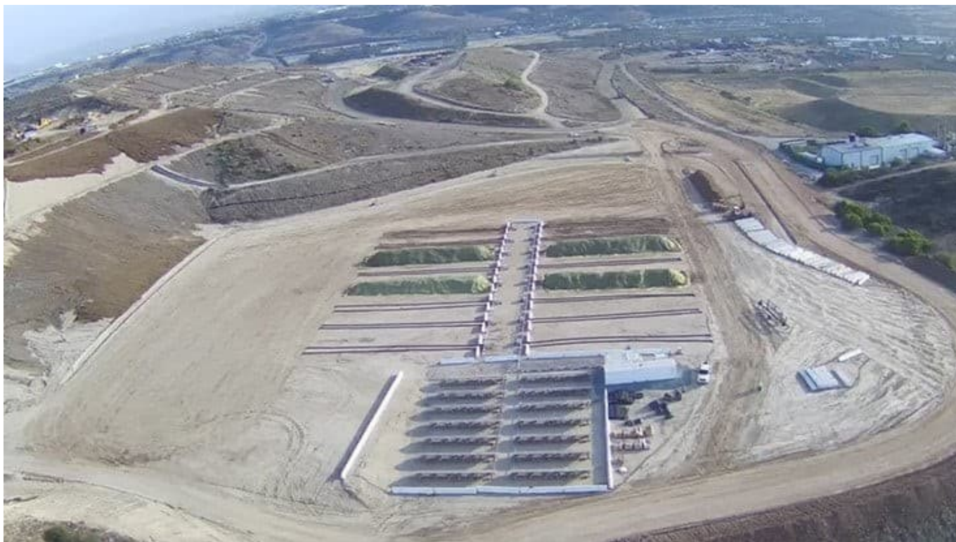
The Otay Compost Facility in Chula Vista, California. Courtesy of Republic Services
