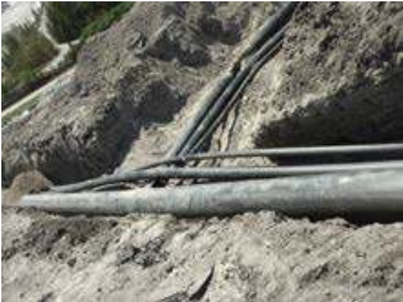
Lateral gas header, condensate force main, and compressed air line involved in final cover construction.
