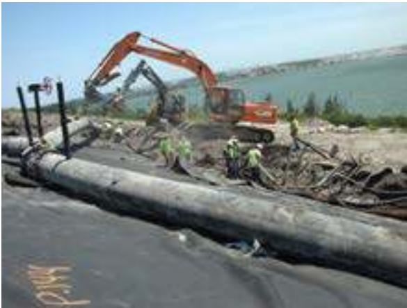
Positioning existing large and small pipes above a new final cover geomembrane.
