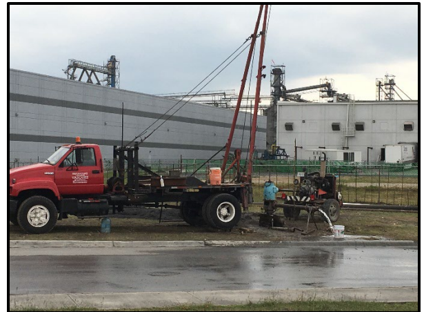
Conducting a pumping test at an Industrial Park to determine the well's extraction rate.
